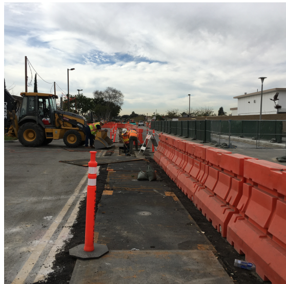
Installation of new domestic waterline at Phase 2
