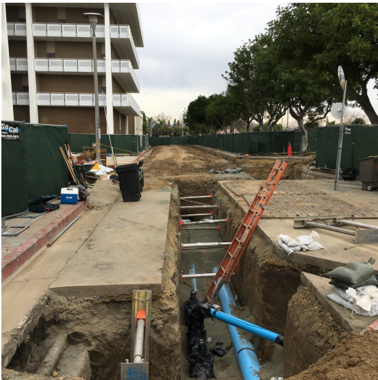
Installation of new domestic waterline at Phase 1
